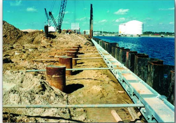
Project: Lake Charles Harbor & Port Improvements Contractor: Cajun Contractors Location: Louisiana
