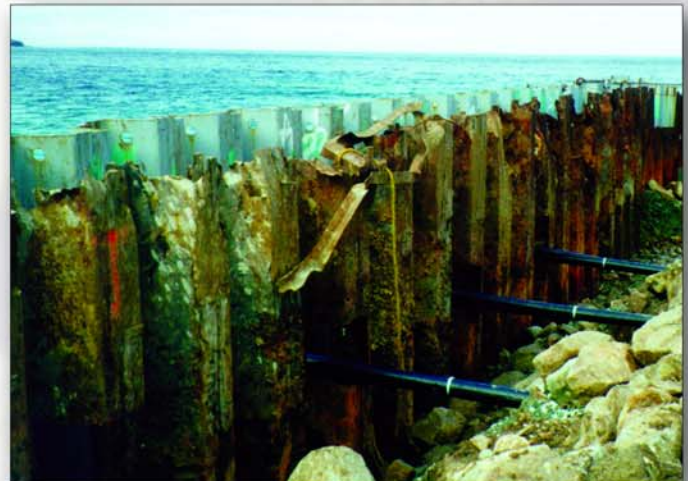
Project: San Clemente Island, Wilson Cove Pier Contractor: American Pacific Marine Location: San Diego, CA
