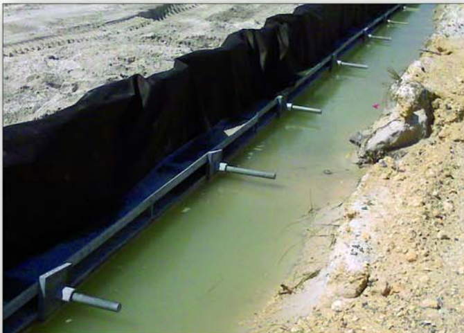
Project: Eglin Air Force Base Contractor: C.W. Roberts Contracting & Contech Construction Products Location: Destin, FL
