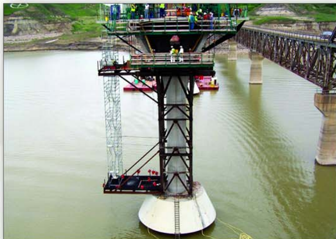
Project: 4 Bears Bridge PT Contractor: VStructural Location: New Town, ND
