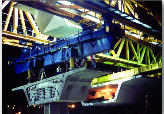
Project: Spaghetti Bowl Contractor: Walter & SCI Construction Location: Las Vegas, NV
