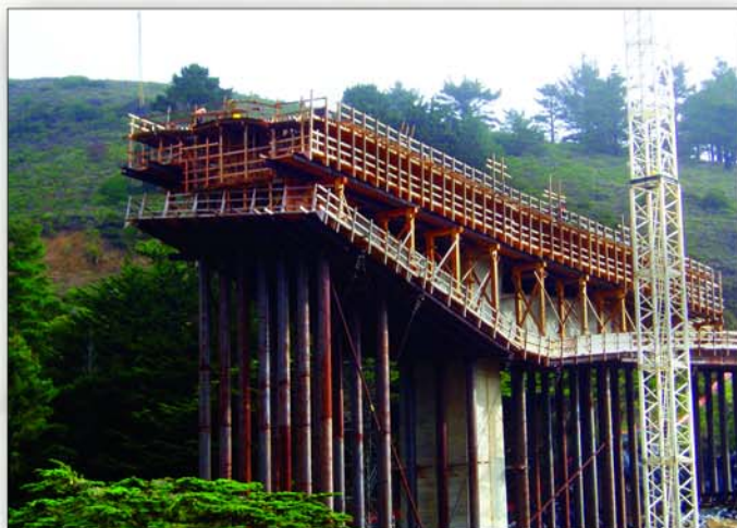
Project: Devil's Slide Bridge Contractor: Disney Construction Post-Tensioning Supplier: Schwager Davis, Inc. Location: Pacifica, CA
