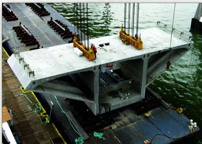
Project Name: San Francisco - Oakland East Bay Skyway Bridge Designer: T.Y. Lin / Moffet & Nichol, JV Contractor: Kiewit / FCI / Manson, JV Post-Tensioning Supplier: Schwager Davis, Inc.
