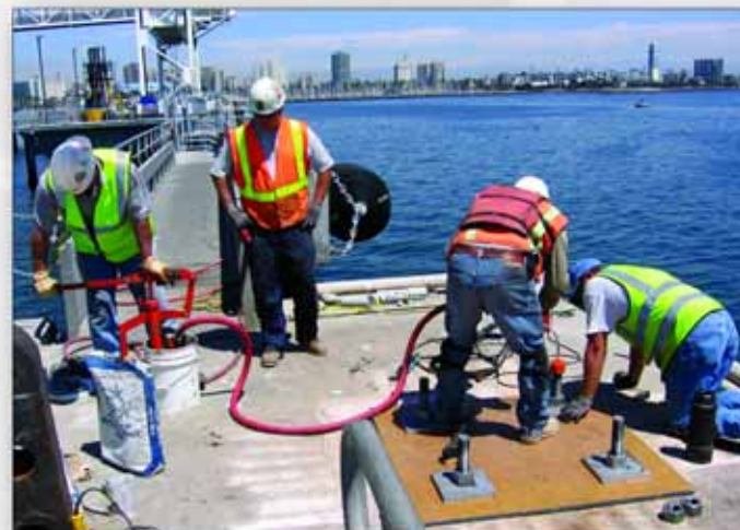
Project: Long Beach Cruise Terminal Designer: CH2M Hill Contractor WW Stevenson Location: Long Beach, CA
