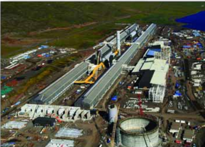
Project: Fjarðaal Smelting Plant Contractor: Bechtel Overseas Corp. Location: Iceland
