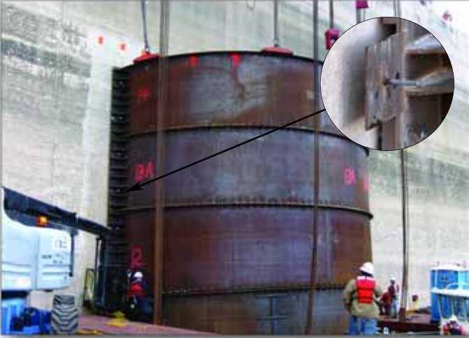
Project: San Vicente Dam Raising Contractor: Barnard Construction Location: San Diego, CA
