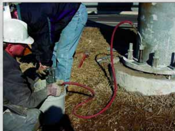
Grouting a Solid Bar Spin-Lock
