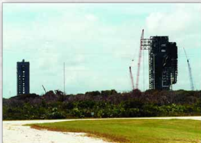
Project: Cape Canaveral Launch Site Contractor: Bechtel National Location: Cape Canaveral, FL
