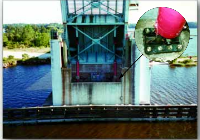
Project: Popp's Ferry Bridge Rehab Contractor: Coastal Marine Contractors Location: Biloxi, MS
