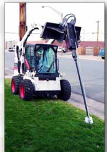
Skid Steer Installation using Shank Adapter attached to Drive Steel
