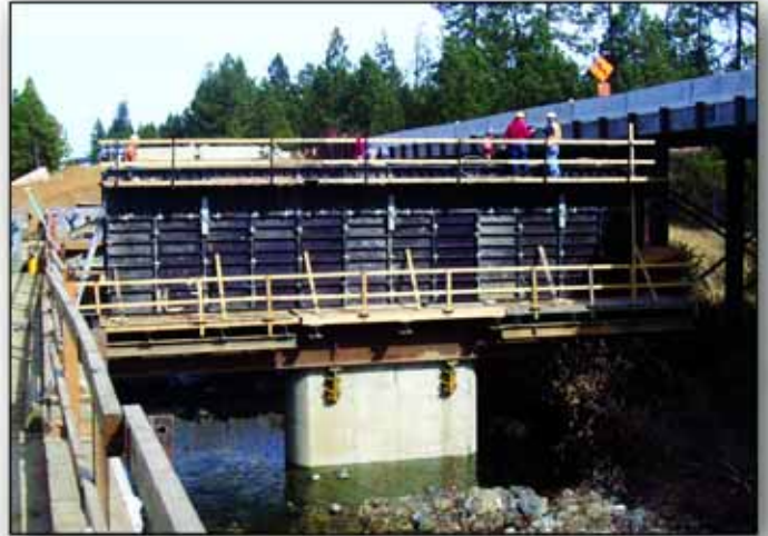
Project: Illinois River Bridge Replacement Contractor: Hamilton Construction Company Location: Cave Junction, OR
